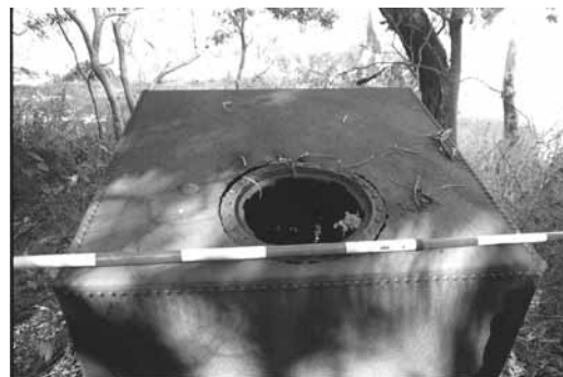
FIG. 11. Water tanks, Friday Island.
